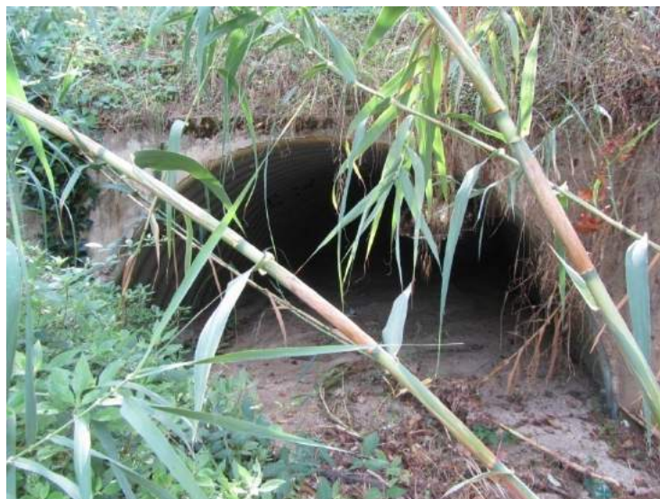
Figura 39. IN_02. Estructura IN_02, torrent Innominat( x=458,444.34 / y=4,602,931.72 )
