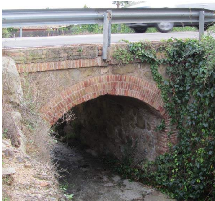
Figura 40. IN_03. Estructura IN_03, torrent Innominat(x=458,454.34 / y=4,602,869.72)
