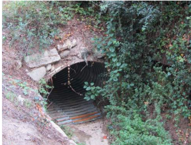
Figura 38. IN_01. Estructura IN_01, torrent Innominat ( x= 458,418.34 / y=4,603,123.72 )
